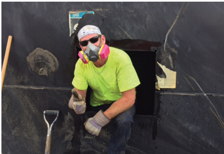
Keller Colley, senior EH&S compliance administrator, cleans out an underground storage fuel tank for disposal. Discarded tanks are frequently sold to scrap yards.
